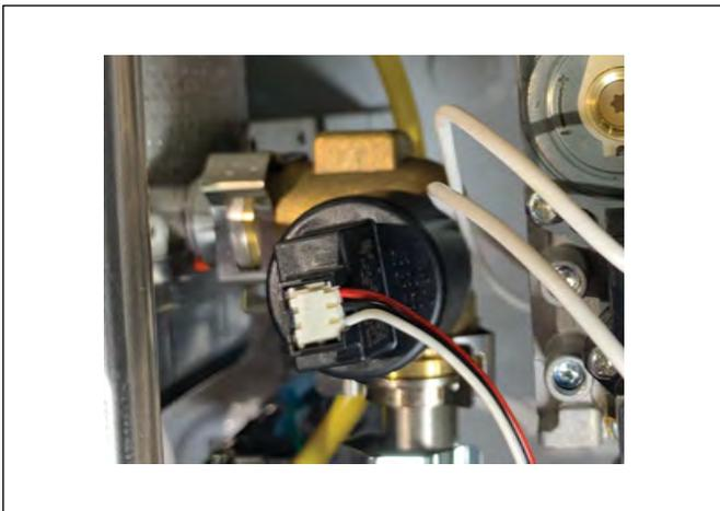
Figure 79 Pressure Sensor
